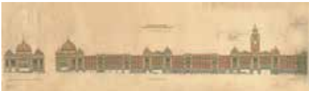
IMAGE 2 Coloured Image of the Flinders Street Elevation ~ 1905
